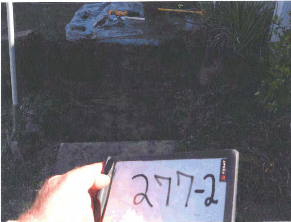
Picture 4: Excavation for UST 277Birch-2.
